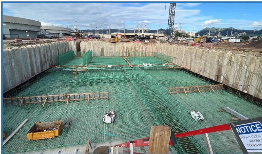
Some of Paul and his crews' excellent, and complex, work.
