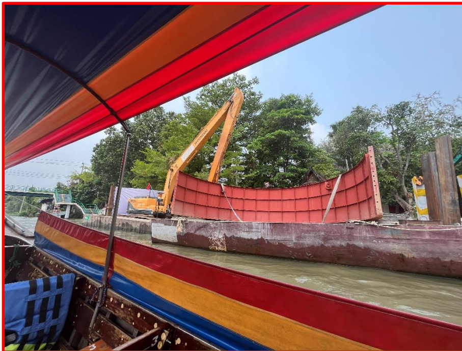
Half of the cofferdam cans I saw along the canals.
