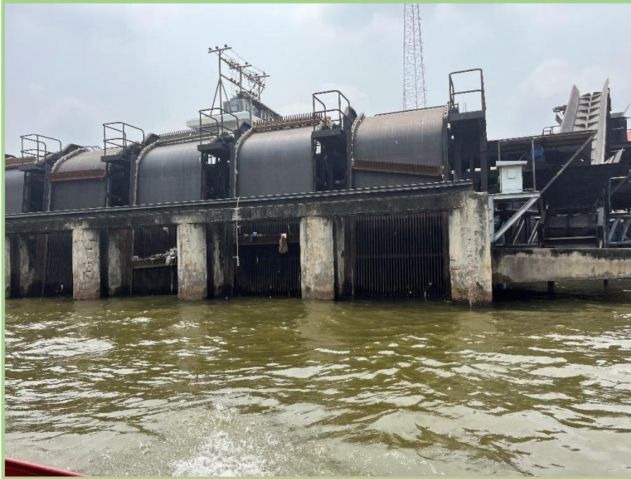
Bar screens to collect river debris. They weren't operating.
