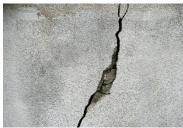
Undesirable cracks that often occur and are not detrimental are usually of a hairline width and occur from the curing process when water has left the concrete too early. These are usually not associated with structural issues.
